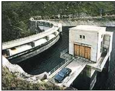
Img 2.4.5 Arch Dam
