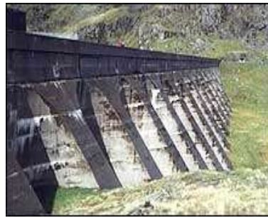
Img 2.4.6 Buttress Dam
