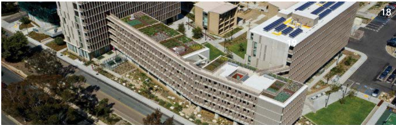
AERIAL SHOWING GREEN ROOF AND LANDSCAPE
