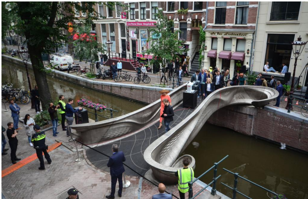
Figure 6 World's First 3D-printed steel bridge in Amsterdam (Parkes, 2021)
