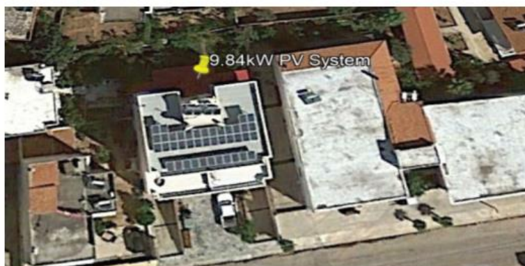
Figure 1. Overview of the PV power plant [10]
