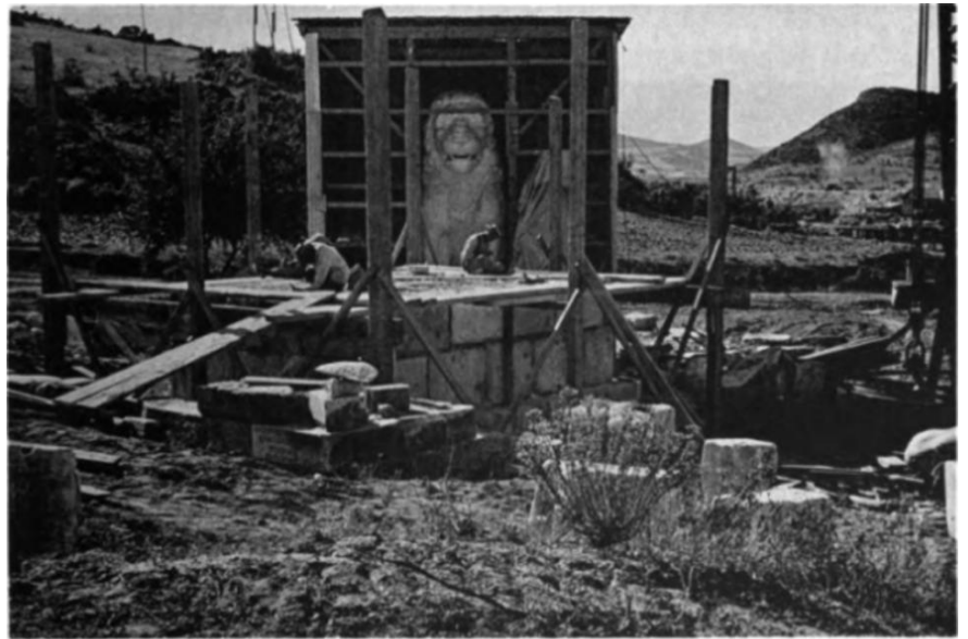
FIG. 12. View of Base during Reconstruction, Plaster Model in Rear.
