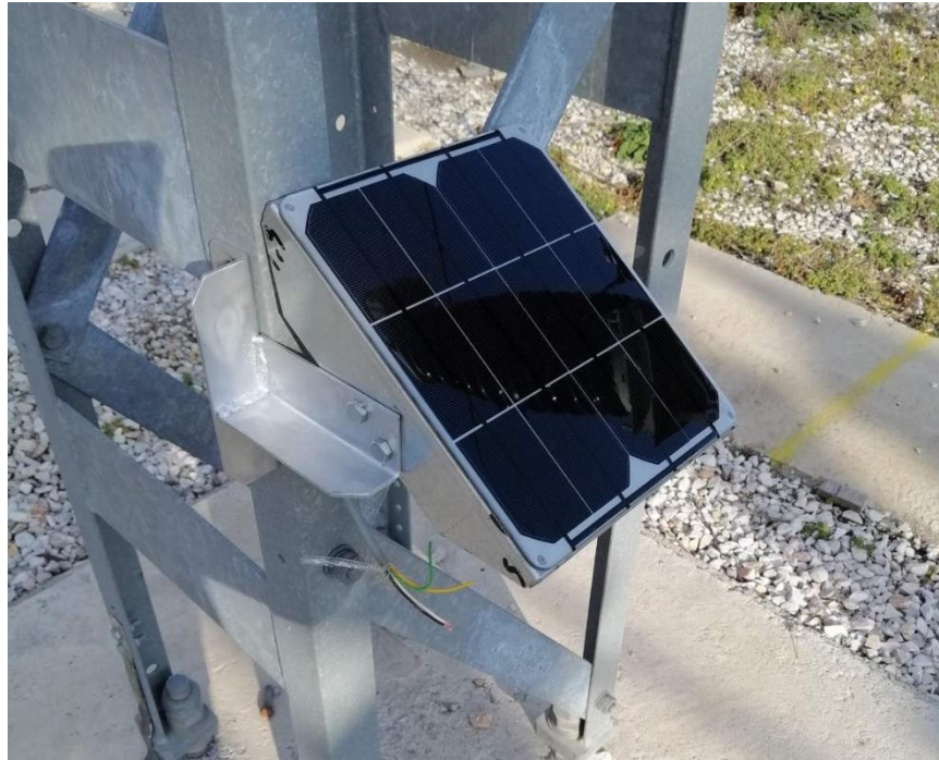
Figure 13 - PV Panel Installation
