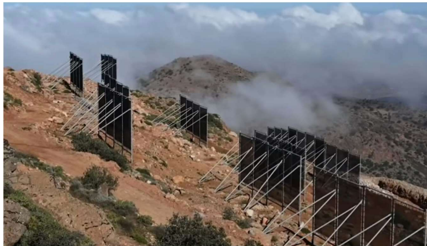
Image 10 Cloud fisher, fog nets (Floating springs, Harvesting drinking water with fog nets, n.d.)
