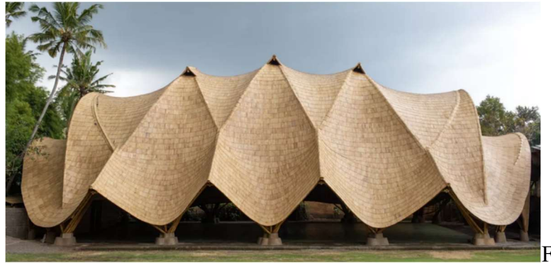
Image 32 The Arc, an educational building at Green School in Bali, with its undulating bamboo roof (Stathaki, 2021)
