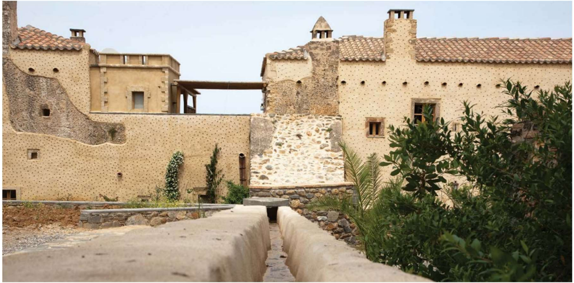
Image 16 The successive phases of construction are rendered visible in contrasting stonework and thick plastic facing (Kinsterna Hotel & Spa / Divercity Architects, 2016)
