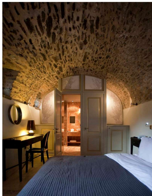
Image 21 Local construction methods and materials capture the atmosphere of the original building. Ceilings feature exposed stone vaults, cypress beams, or traditional woodwork (Kinsterna Hotel & Spa / Divercity Architects, 2016)
