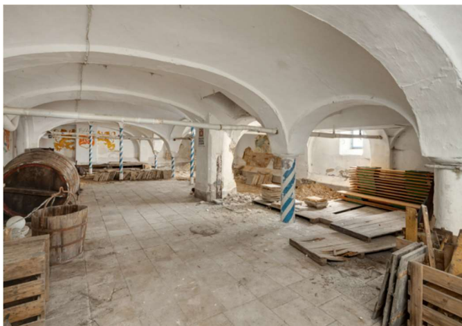
Image 29 Conversion of a Former Brewery to a hotel / KUHLEIN (Conversion of a Former Brewery to a Hotel / KÜHNLEIN Architektur, 2018)
