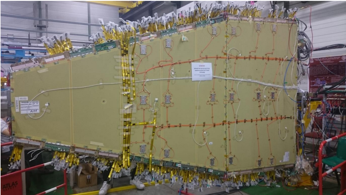
Figure 72: A large MM sector during the installation of electronics.
