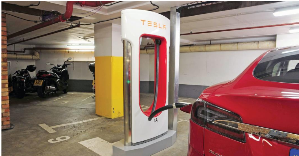
Σχήμα 1.2 Tesla Supercharger with charging potential up to 150 KW
