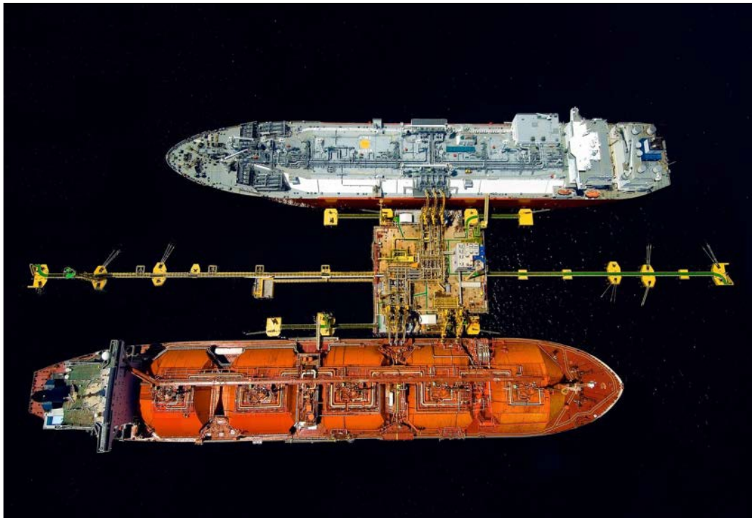
Picture 12: Ship to jetty to FSRU transfer, jetty is equipped with regasification plant [31, p. 20]
