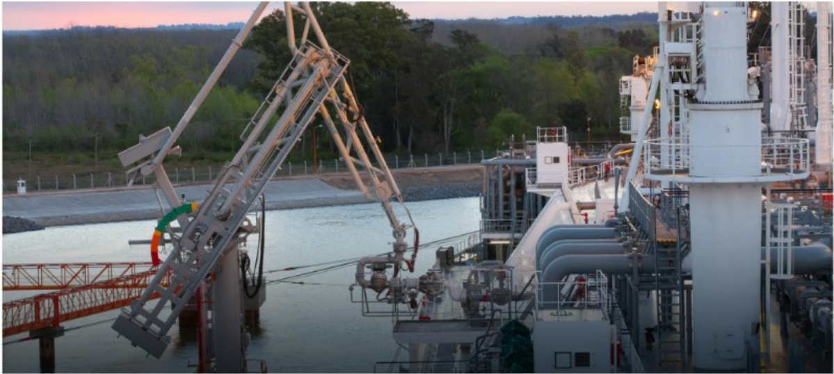
Picture 18: Natural gas is discharged via high-pressure gas offloading arm [53]
