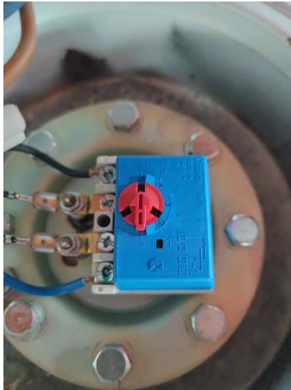
Figure 36: Element Circuit & Temperature Set – Ups
