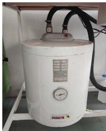
Figure 83: Boiler – Water Heater Placement
