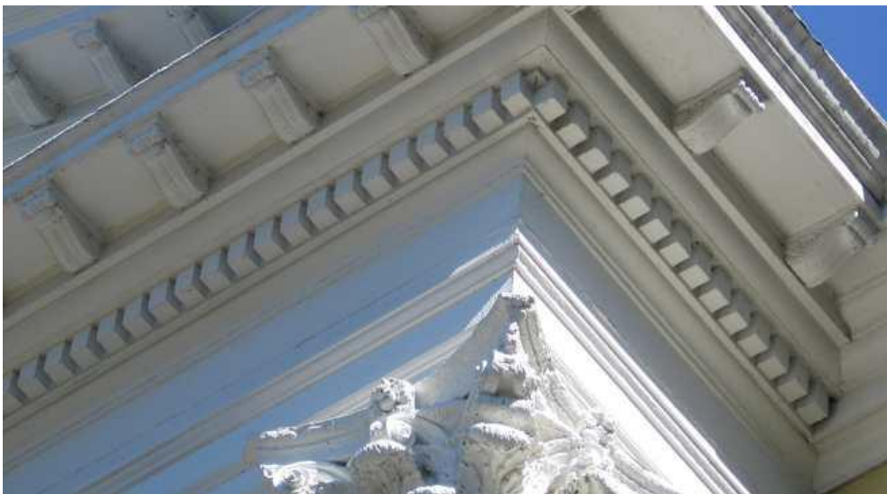
Figure 32, Skeuomorphic pillars in an ancient Greek temple. Note the decorative support beams.
