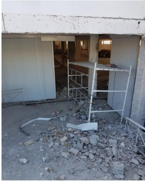
Image 137 Repair work done on the MINOIKI factory at Petrou Ralli Street, 2021
