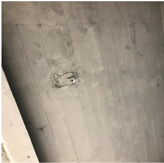
Image 116 Ceiling hook in the building of the former "Nikolopoulos Bros.", 2019
