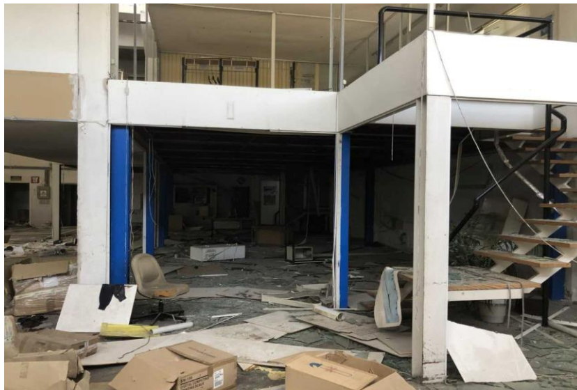
Image 93 Interior of the former BIOSISAL plant at 4 Aristotelous Street, 2020
