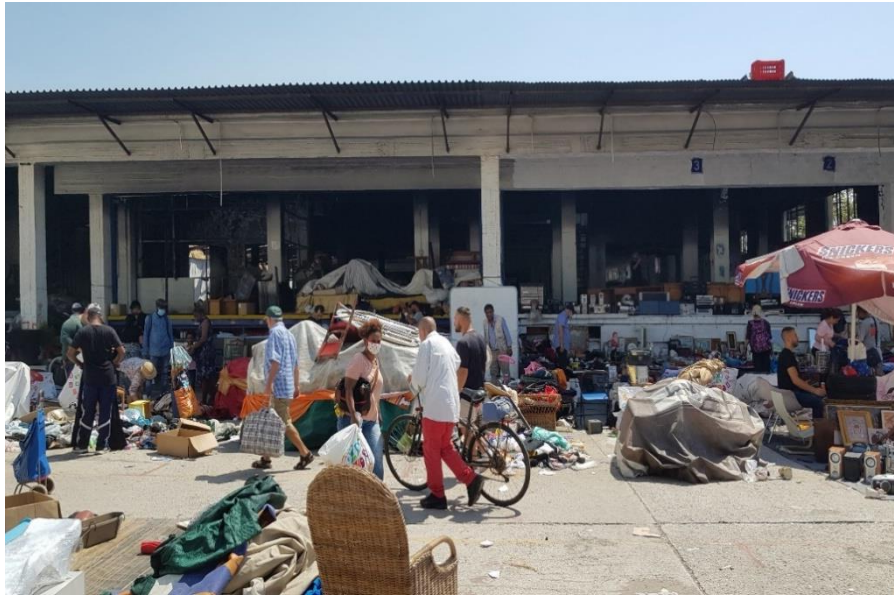
Image 48 Industrial building part of the wastepicker market in the Eleonas, 2022
