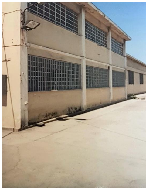
Image 109 View of the former ELVIS plant at Orfeos Steet, 2009
