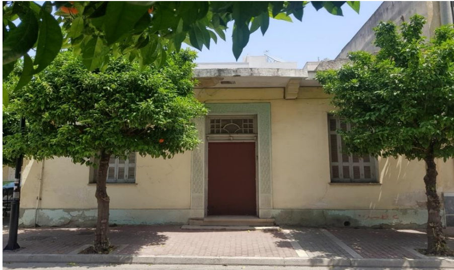
Image 34 Single-storey residence at Diomidous Street in the community of Estavromenos, 2022
