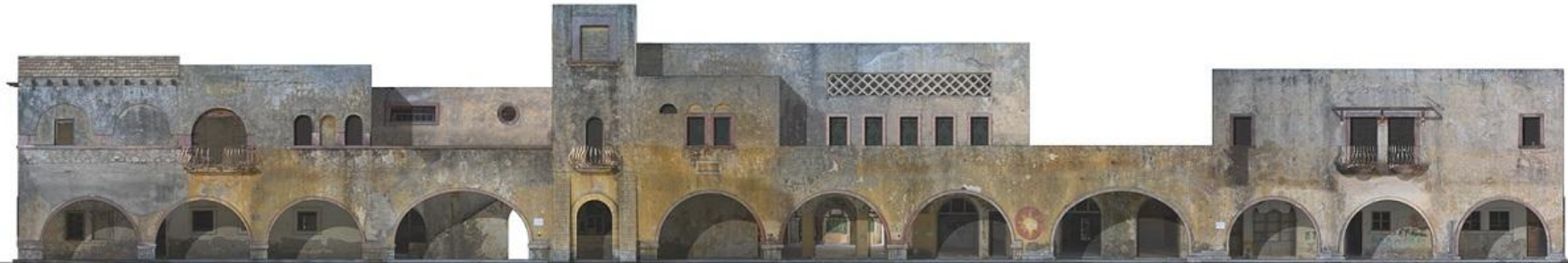
Building 1, Elevation SE, Current situation (2018)
